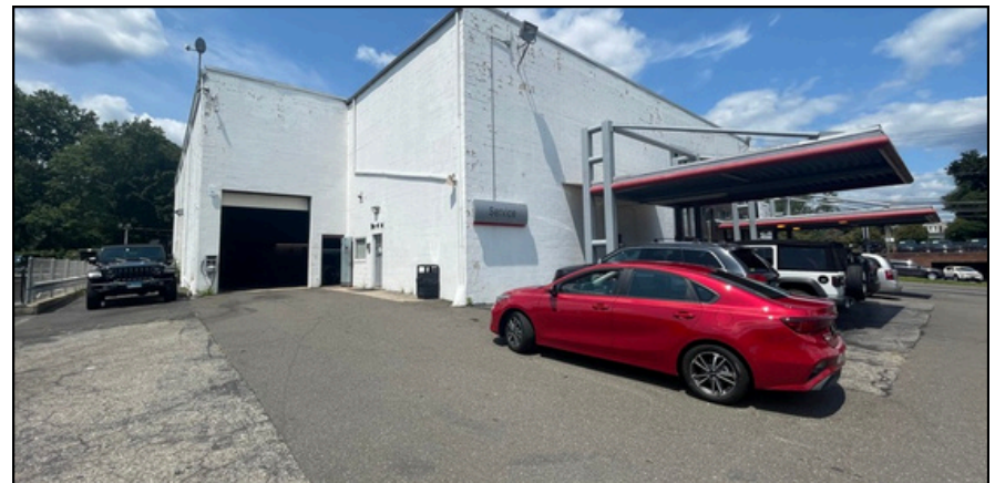
SIDE ENTRANCE TO SERVICE AREA
